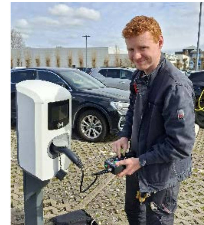
Jonathan Bollens with one of our now 190 charging points in Turnhout.
