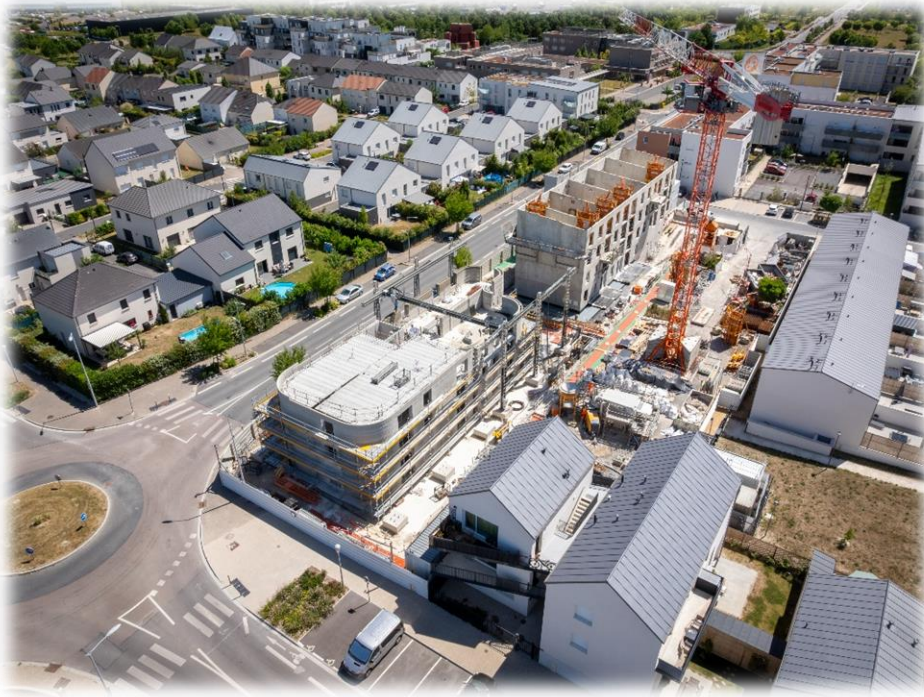
ViliaSprint 2 - ©PERI 3D Construction
