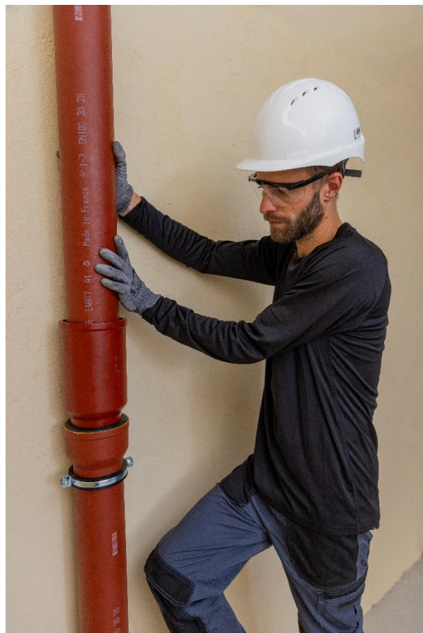
Crédit photos Pam Building
