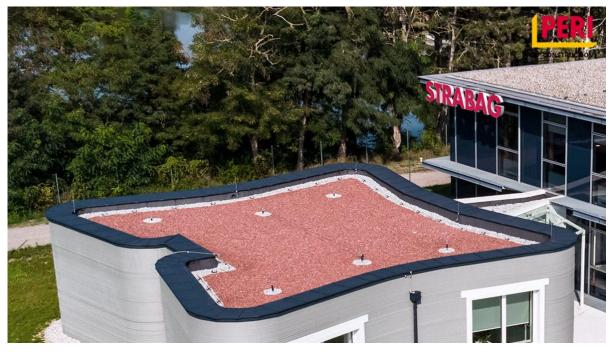
The 125 m2 office extension building printed by PERI with a COBOD BOD2 3D construction printer
