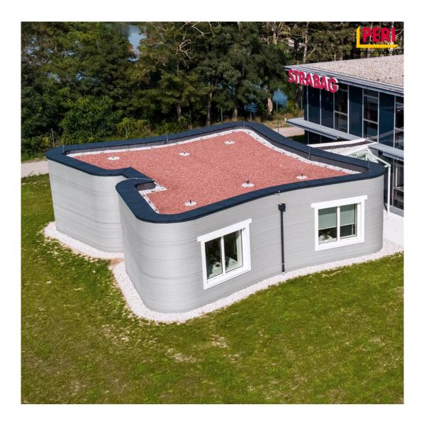
Image caption: The 125 m2 office extension building printed by PERI with a COBOD BOD2 3D construction printer
